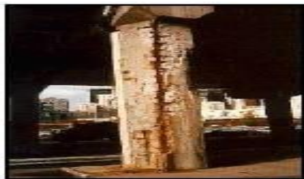
Fig 5.4 : Corrosion in the Steel
