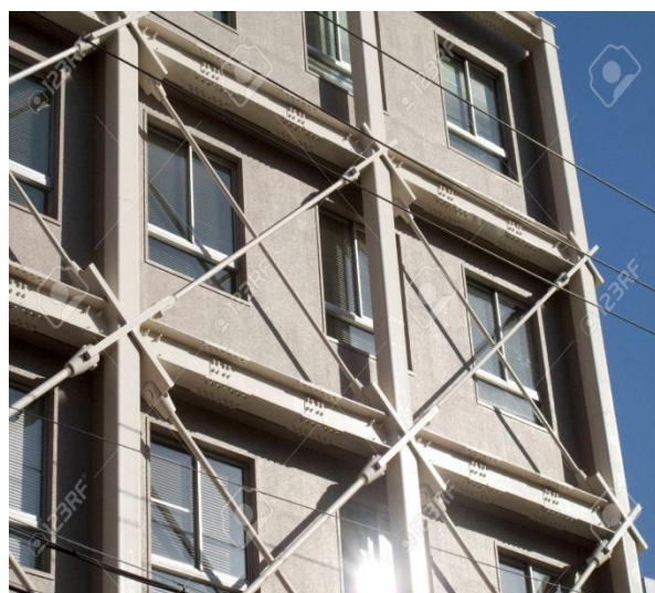
Fig 14.2 Seismic Retrofitting of Building
