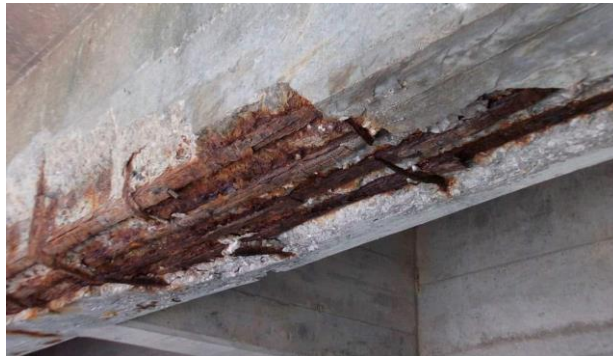
Fig 5.4 : Corrosion in the Steel
